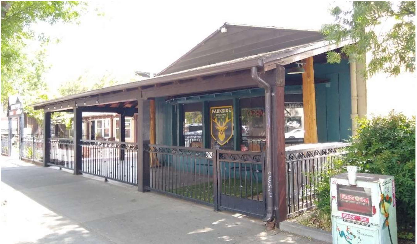
West façade of southern "leg," ESA 2022
