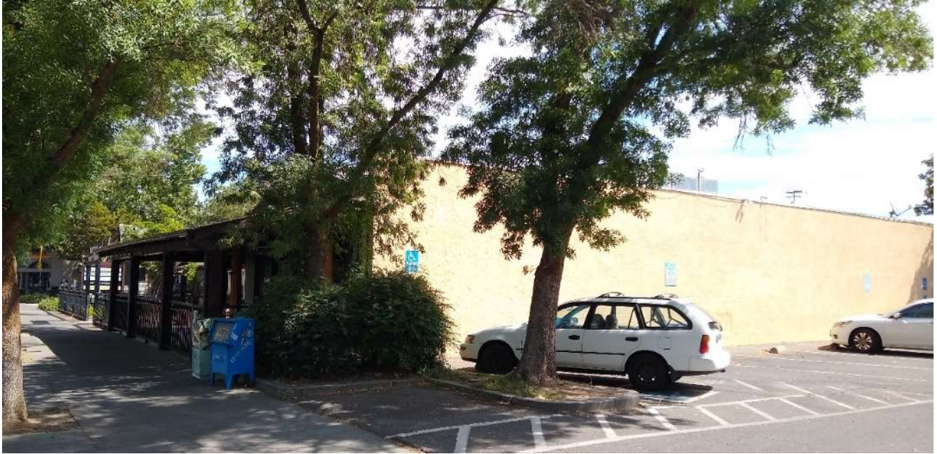
West and south facades of southern "leg" of U-Shaped building, ESA 2022
